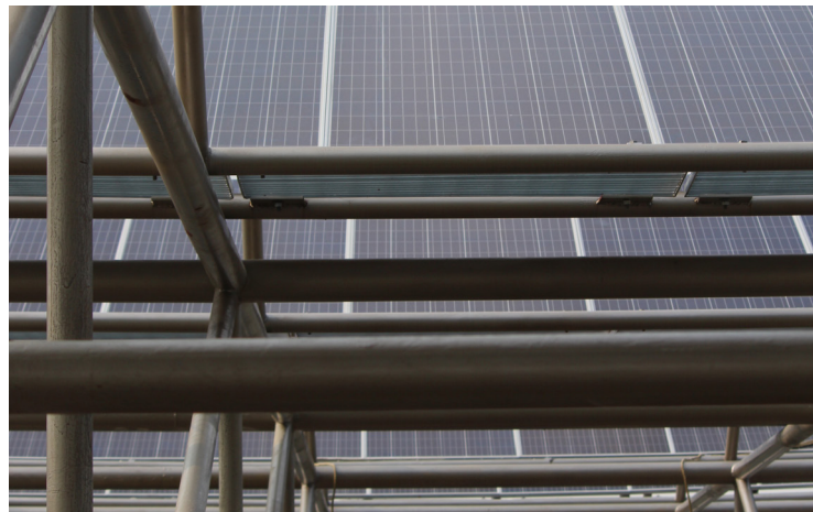
# Solar Panel installation
